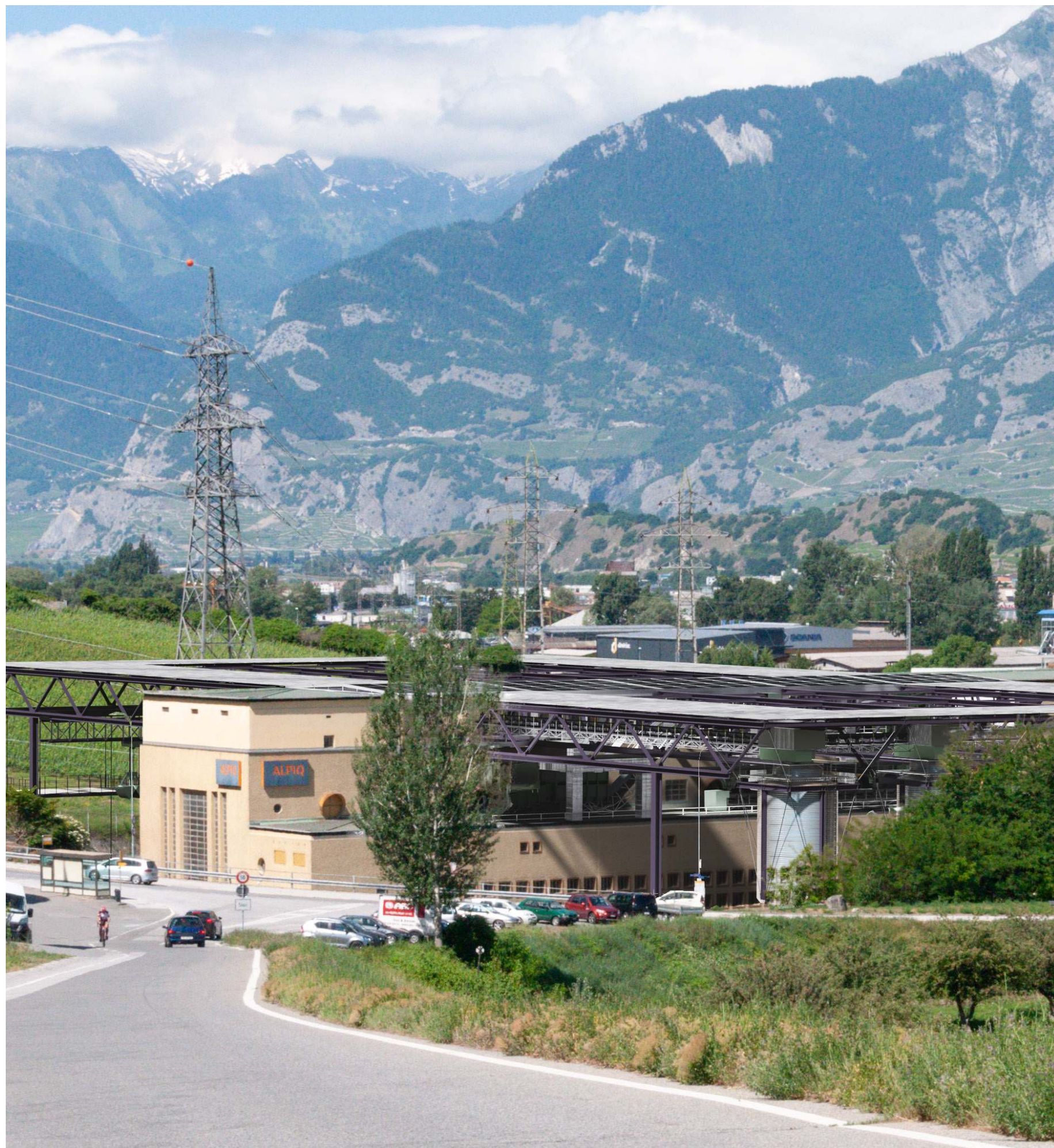
The cultural center gets protection from its industrial cloak which guarantees dust, noise and a stream of trucks
